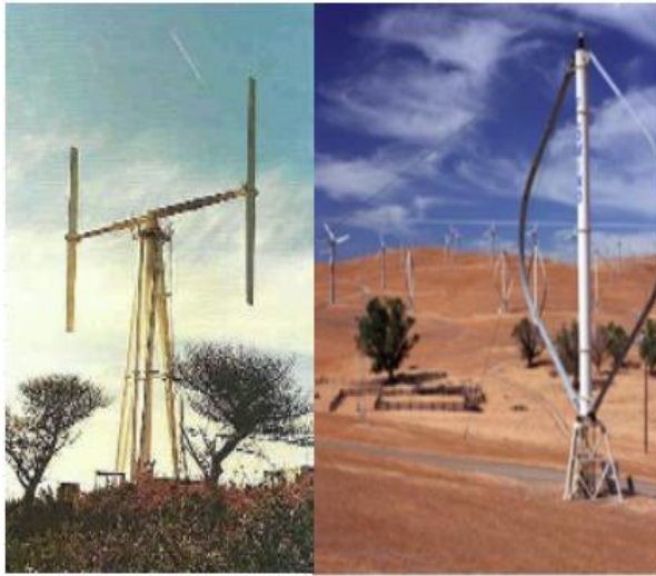
Fig 5. H-Rotor and Darrieus rotor [14]
